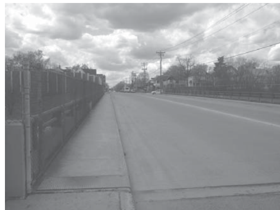
E 38th Street Bridge over 35W
